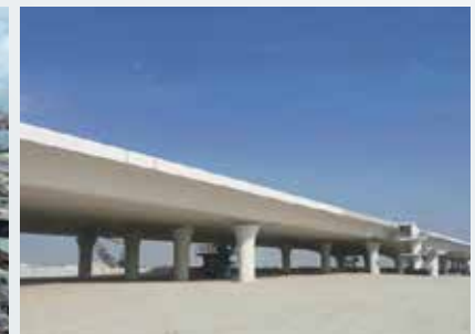
Red Sea Village Development, Kingdom of Saudi Arabia OVM supplied PT system and construction supervision.
