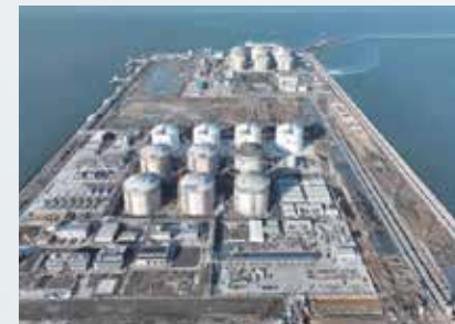
Tianjin LNG Tank Project, China OVM supplied Cryogenic Prestressing system.
