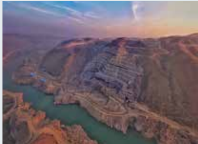
Mohmand Hydropower Project, Pakistan OVM supplied strand tendon (active) anchor system and construction equipment.
