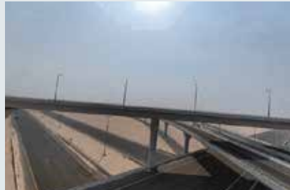
Project of RA 259, Kuwait OVM supplied PT System.
