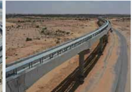
Cairo Monorail project, Egypt OVM supplied PT System.
