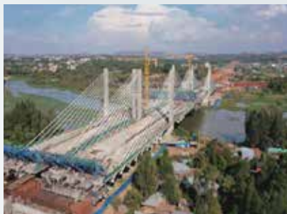
Aby River Bridge, Ethiopia OVM supplied PT system, extradosed stay cable system and construction.
