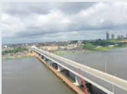
4th bridge of Abidjan, Côte d'Ivoire OVM supplied PT system.
