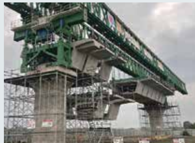
North-South Commuter Railway, Philippines OVM supplied PT system.
