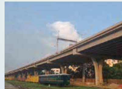
Dhaka Elevated Expressway, Bangladesh OVM supplied PT anchorages and bridge bearings.
