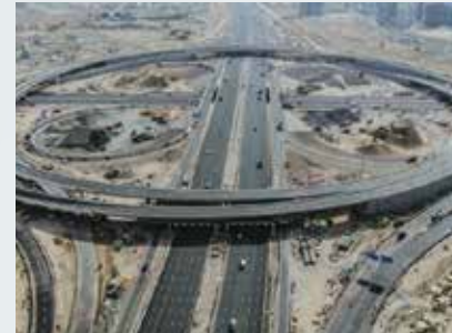
Improvement of EXPO 2020 Roads, Dubai OVM supplied PT System.
