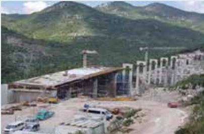
Overpass Preljubovica, Montenegro OVM supplied PT system and equipment.
